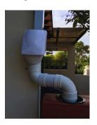
Install the downpipe into the inlet pre-fitted with leaf strainer. Either end can be used.
